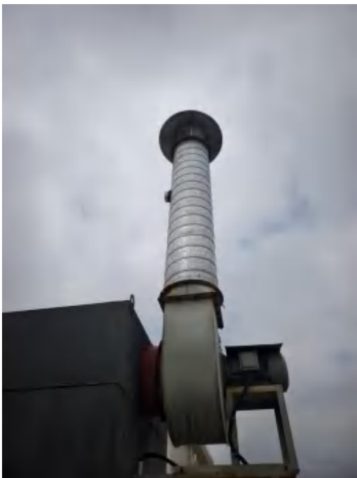
拌料、投料粉尘DA002排气筒照片
